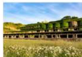
KITAZAWA FLOTATION PLANT
