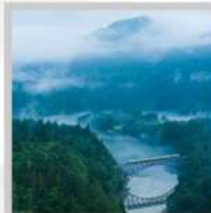
"TADAMI FIRST BRIDGE"
